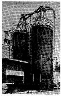
These Permaglas<sup>R</sup> structures have built-in sanitary features. Their glassbonded-to-steel walls fight the many contamination problems faced in handling and storing raw materials and processed products.
